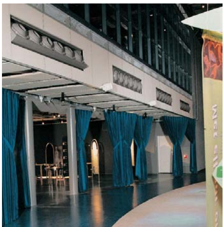
Swivel jet nozzles, type DW-V2, in swivel connection boxes in the 'New Metropolis' science and technology centre, Amsterdam / NL
