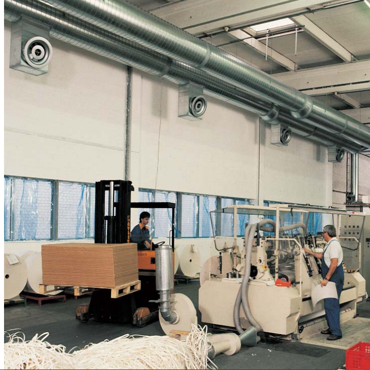
Swivel jet outlet, type SW, in a manufacturing hall of the paper mill 'Sihl GmbH' in Düren / D
