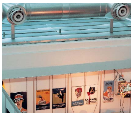
Swivel jet outlet, type SW, at the 'Design Center Linz', Linz / A
