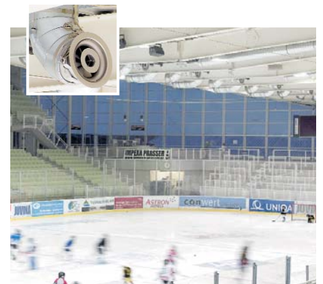
Swivel jet outlet, type SW, in the Albert Schultz Ice Skating Hall, Vienna / A
