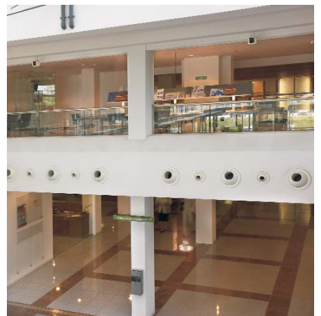
Swivel jet nozzles, type DW-V2, at the 'Atrium medisch centrum', Heerlen / NL
