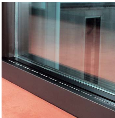
Window air curtain unit, type FSG, in an office of the Dresdner Bank AG in Frankfurt am Main / D
