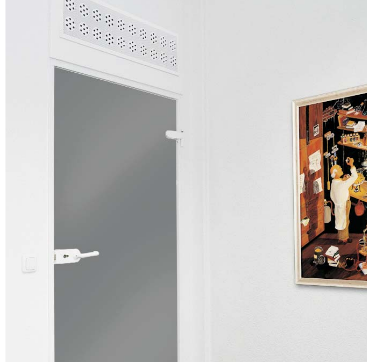
Broad multiplex outlet, type BF, in an office
