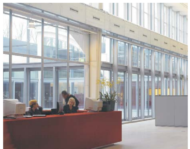
Multiplex outlet, type FA-VT, single-row design, in the entrance hall of the Ogilvy Marketing Agency, Amsterdam / NL
