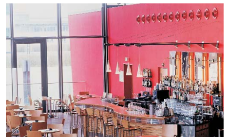
Swivel jet nozzle, type DW-V2, in the restaurant of the multiplex 'Filmpalast-am-ZKM' in Karlsruhe / D
